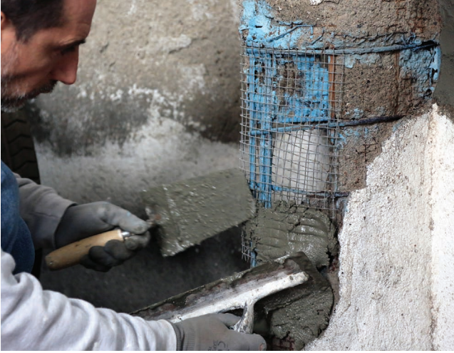
Figure 18. Preserving the Magliana warehouse ferroconcrete wall, 2013, © Sixxi
