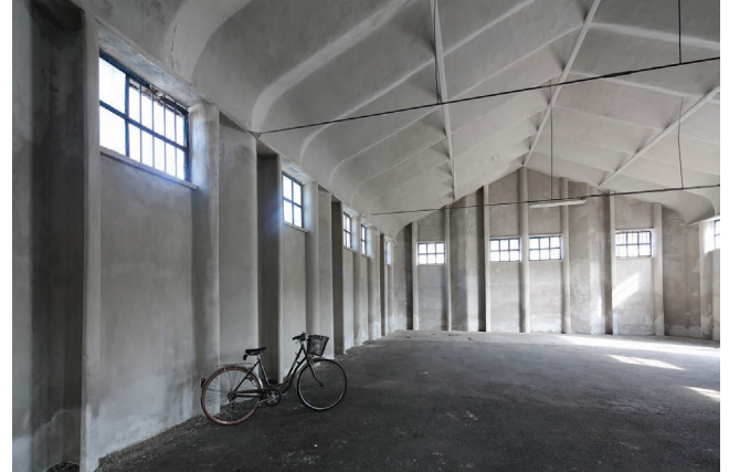
Figure 20. The Magliana warehouse after the ferroconcrete restoration works, 2013, © Sixxi
