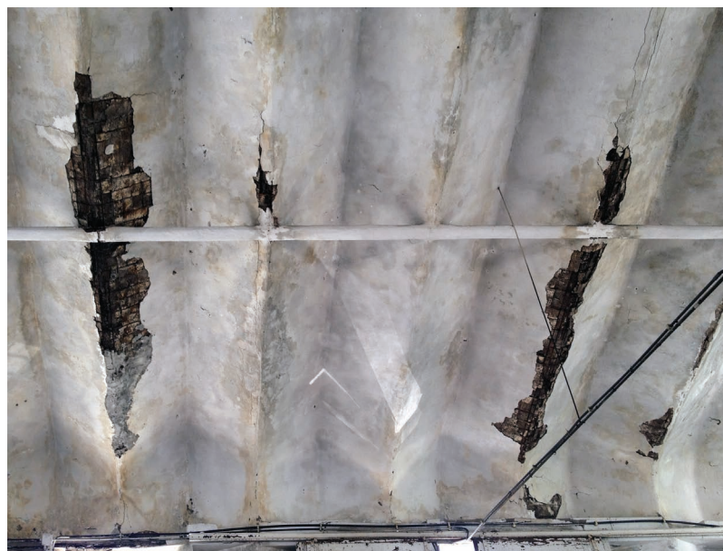
Figure 17. The Magliana warehouse roof before the restoration works, 2012, © Sixxi
