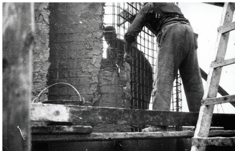
Figure 7. Workers building the Magliana warehouse walls, 1944–1945 (reproduced by agreement of Centro Archivi Maxxi, Rome).
