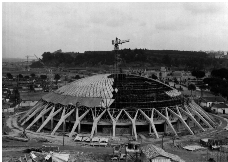
Figure 10. The Palazzetto dello Sport under construction, 1957 (reproduced by agreement of Coni Historical Archive, Rome)
