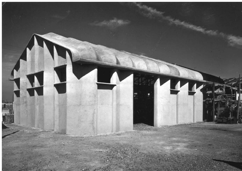
Figure 3. The Magliana warehouse under construction, 1945 (reproduced by agreement of Centro Archivi Maxxi, Rome)
