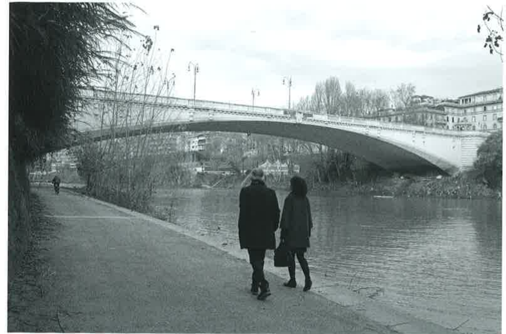
Figure 2. Risorgimento bridge over the Tiber, Rome. F. Hennebique, G.A. Porcheddu, 1909-11. Photo: Sergio Poretti.
