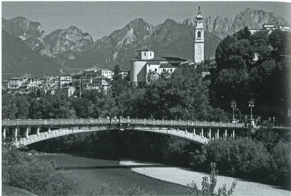
Figure 3. Victory Bridge over the river Piave, Belluno. E. Miozzi, 1925-26. Photo: Sergio Poretti.
