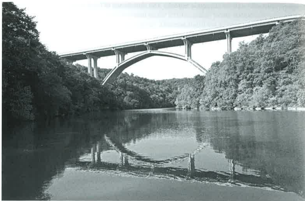
Figure 6. "G. Romita" bridge over the Arno, Highway of the Sun, Levane. S. Zorzi, 1962-64. Photo: Sergio Poretti.
