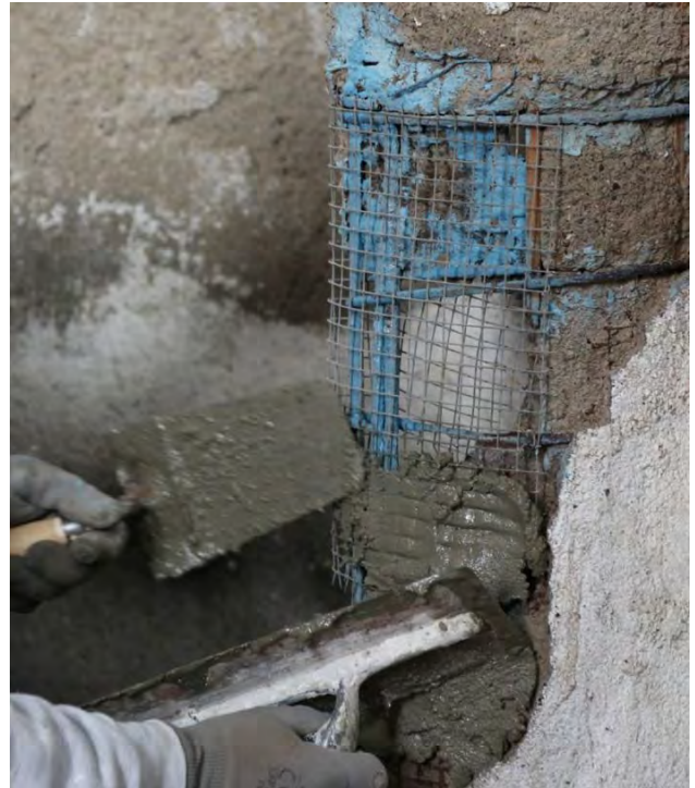
Fig. 6. Magliana Warehouse. Restoration works, 2013 (Photo Sergio Poretti, SIXXI Project).
