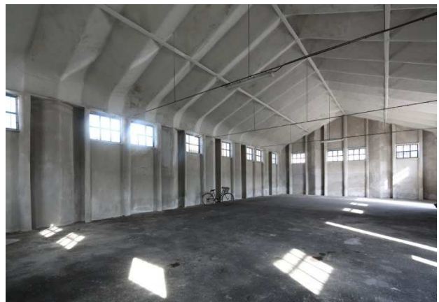
Figure 7. Magliana Warehouse. Interior after restoration works, 2013
